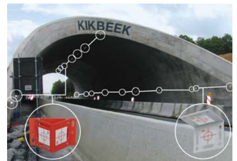
Construction of Ecluduct Belgium
