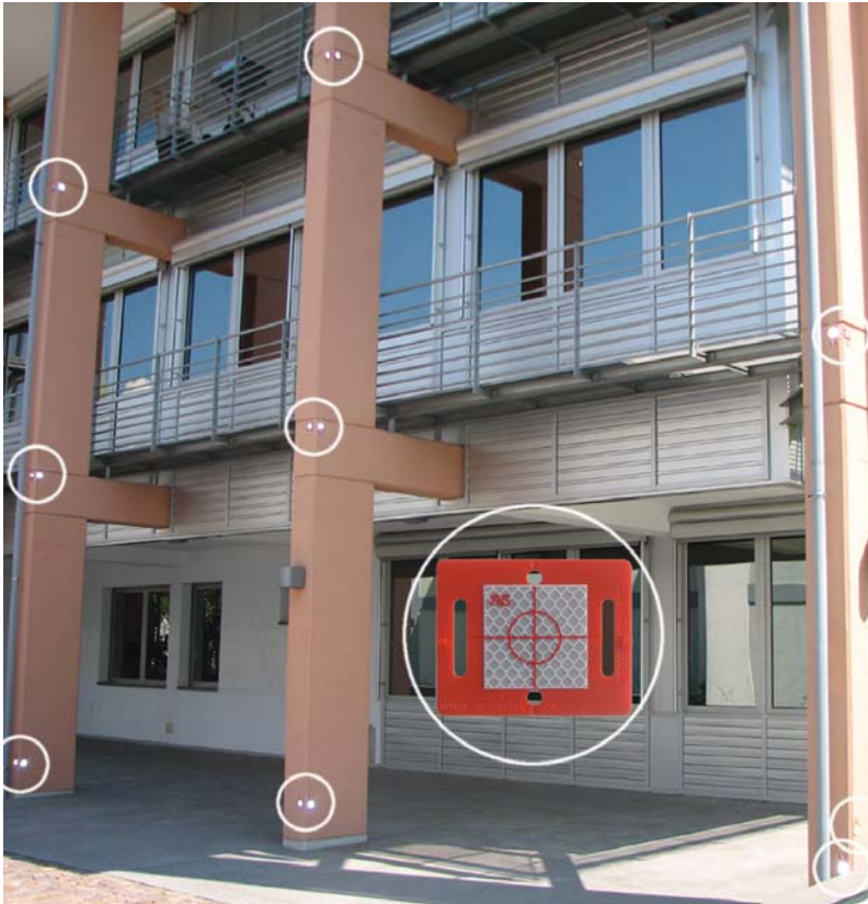
Monitoring of a façade using RS60r
