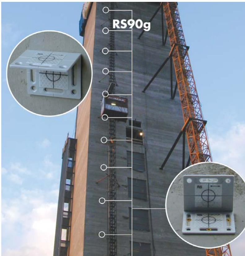
Climbing formwork with RS90g
