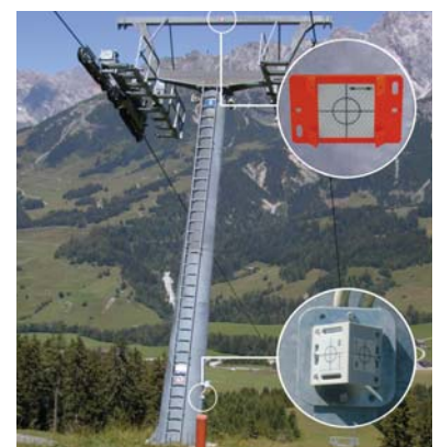
Monitoring of ski lift supports using RSAKZ6r and RSAM80g
