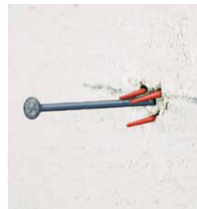
Elastic "stubs" for securing the surveyed measurements are securely marked until plastering work is completed.
